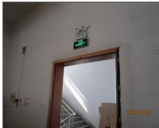
Photo of fire safety equipment fire alarm and fire exit sign and emergency light.JPG
